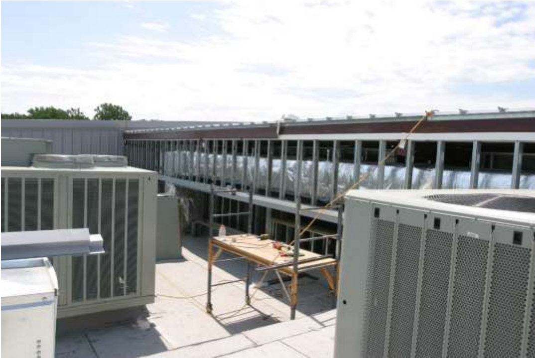
Construction photo from 6/17/2008
