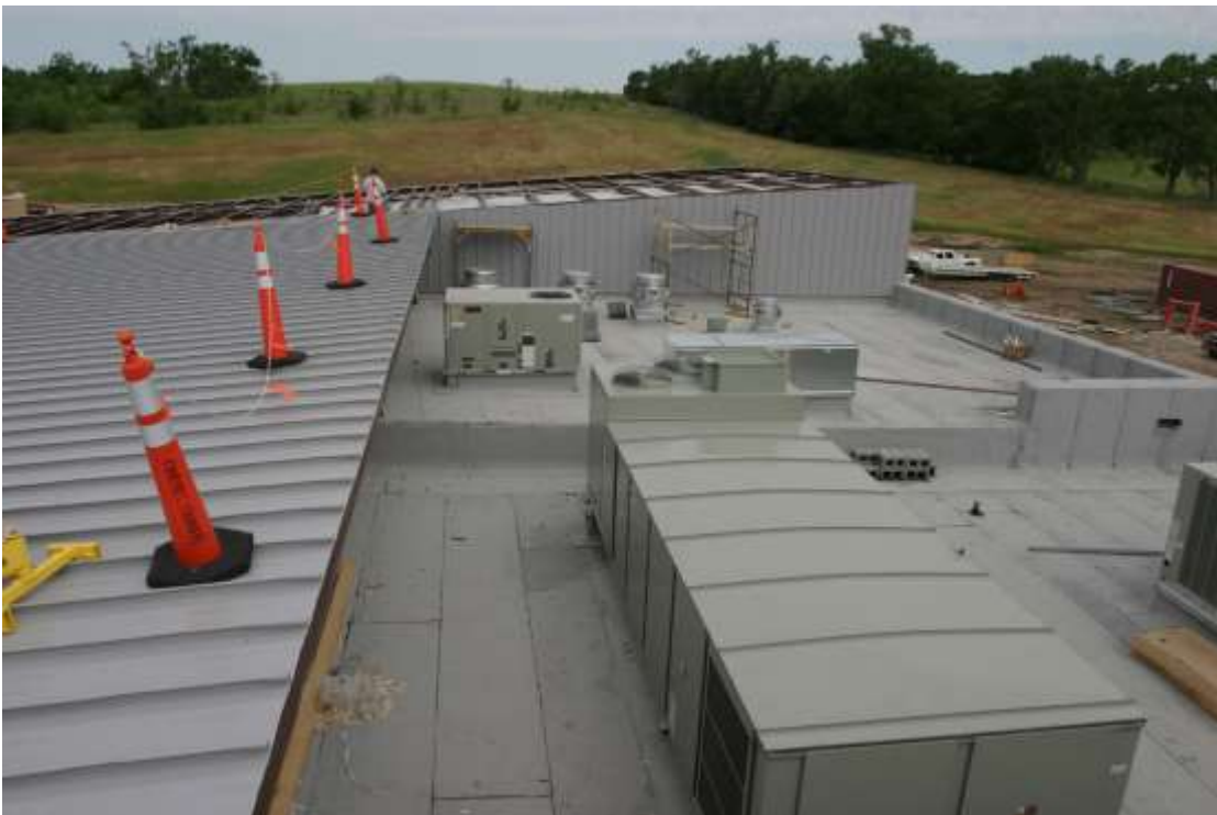
Construction photo showing equipment on kitchen roof.
