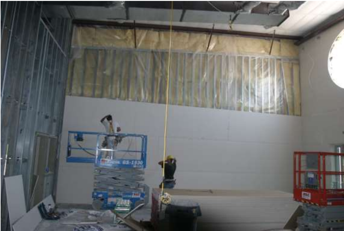
Construction photo from 7/21 2008.
